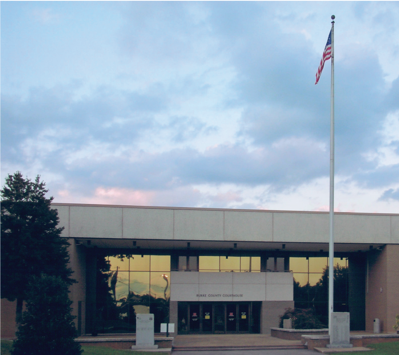
Burke County Courthouse ▼
