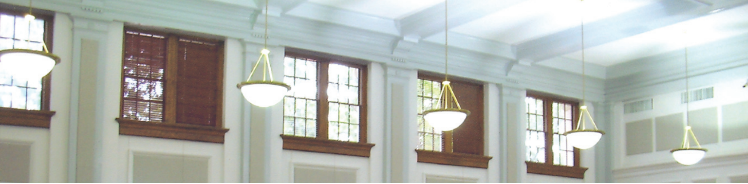
▲ Moore County Courthouse
