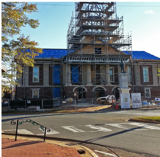
photo courtesy of Hobbs Architects
