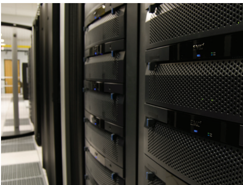
A small-scale server farm is the hub for network connectivity and data storage, and retrieval for court-related information.
